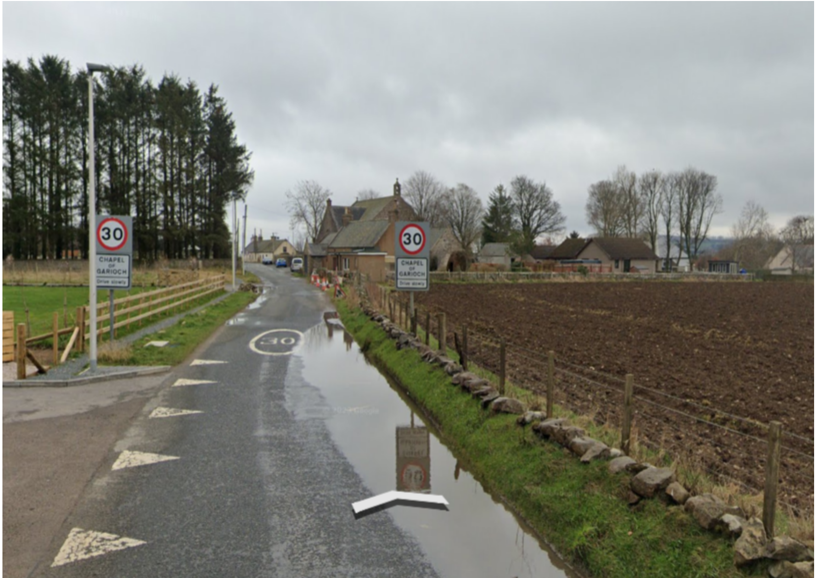
Approaching the site from the east
